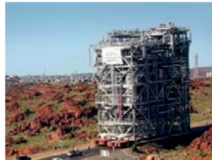
Figure 2: The world's first preassembled LNG plant by Worley Parsons, North West Shelf, Australia: an extreme example of 3rd generation modularisation.
